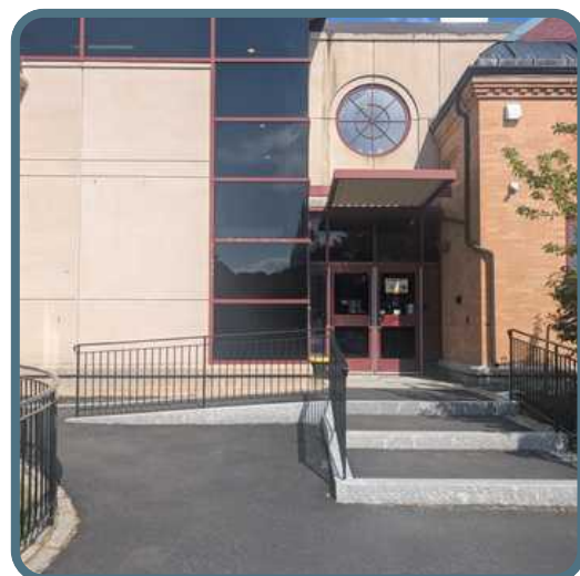
Improved accessibility entrance
